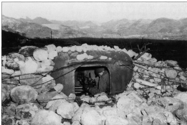
ABOVE A US soldier examines the internal workings of a captured MG Panzernest. It has been covered in rocks for added protection and camouflage. Just visible in the right foreground is a German mess tin. (US National Archives, 187023)
