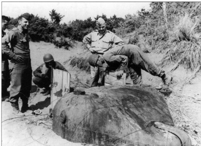
ABOVE American soldiers inspect an MG Panzernest that has been installed to cover one of the many beaches. The shield at the front, which was used to protect the aperture when the machine gun was not in use, is clearly visible as are the openings at the side that were used for the axle and for ventilation. The two periscopes at the top can also be seen. (US National Archives, 192342)
