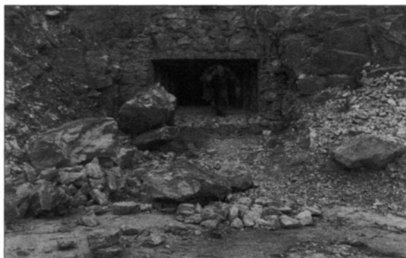
BELOW An Allied soldier emerges through the embrasure of a gun position that was hewn in the side of a mountain. The position covered the road that ran down the Serchio Valley near Galliciano. The opening was camouflaged with stone cladding. (Imperial War Museum, NA21202)
