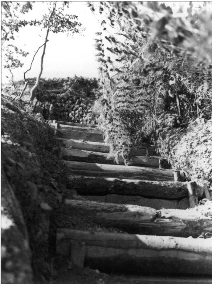
BELOW A flight of steps constructed from logs held in place by wooden pegs. They led to a German position in the Gothic Line. Camouflage nets, that would have prevented Allied planes spotting the position, hang limply at the side. (US National Archives, 359053)
