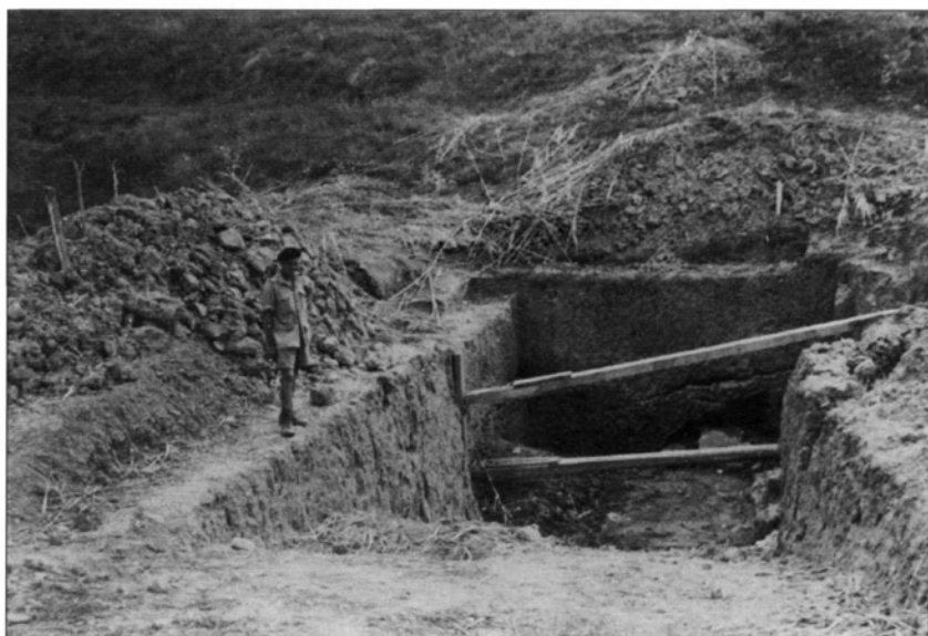
RIGHT An excavation ready to accommodate the upper and lower boxes for a Panther turret. The base section would have been manoeuvred down the inclined plane, a technique used when no lifting gear was available. (J. Plowman)
