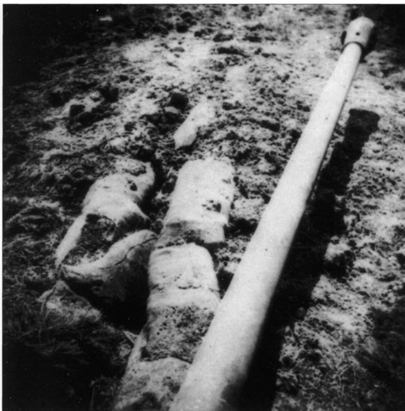
LEFT A Panther turret gun barrel showing the sandbag channel that it was lowered into to either hide its distinctive shadow from aerial observation or to reduce the strain on the elevating gear. (Imperial War Museum, HU60080)
