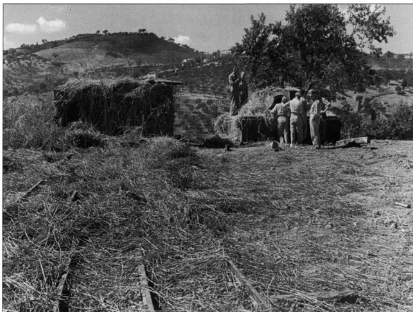
RIGHT A Panther turret and steel shelter ready for installation. In the foreground are the rails on which the lower box, which formed the crew's living quarters, was moved into place. The two sections have been covered in hay in an effort to camouflage them. (Imperial War Museum, NA18343)
