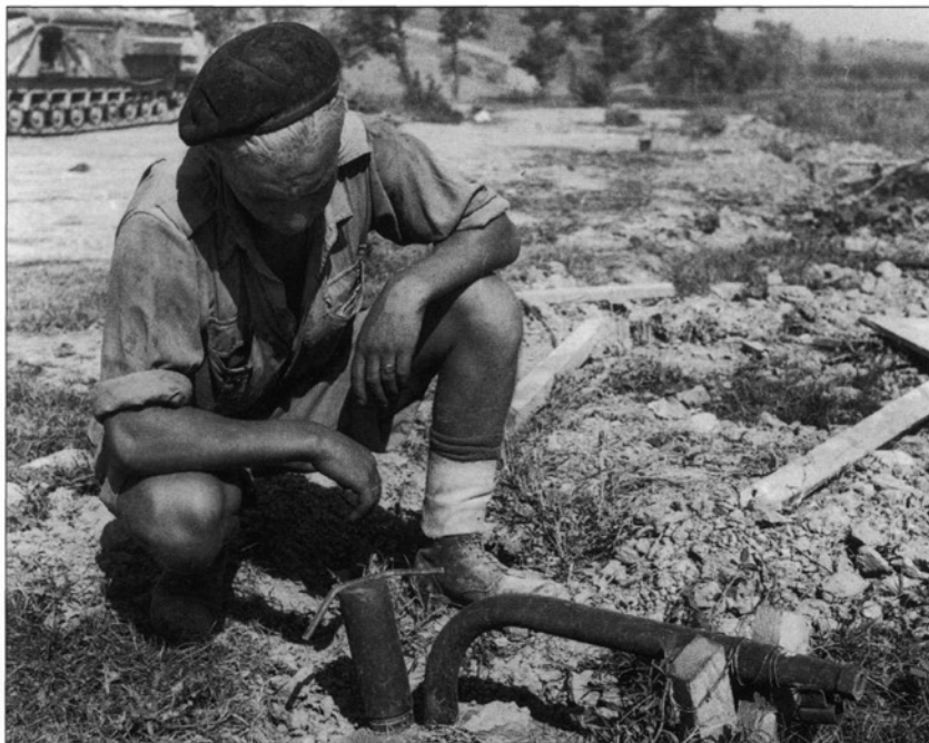
LEFT An Allied soldier inspects one of the flamethrowers that were used in the Gothic Line. The fuel tank of the Abwehrflammenwerfer 42 was buried in the ground so that only the nozzle was visible. They were often used in groups and when triggered would project a jet of flame for some 50m. (Imperial War Museum, NA 18338)
