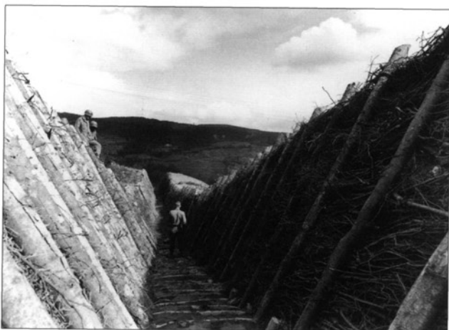
BELOW American soldiers inspect a section of the anti-tank ditch of the Gothic Line. The technique for revetting the sides is clearly evident with uprights held in place by wire securing the brushwood behind. (US National Archives, 1946245)
