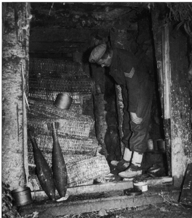
ABOVE In order to safely store their ammunition for the weapons employed along the Gothic Line the Germans blasted a number of caves in the mountains. This cave was located near Castiglione Dei Pepoli. It was 5m deep and strengthened with timber props. It was used to house mortar rounds, as shown, and 170mm artillery shells. (Imperial War Museum, NA19204)
