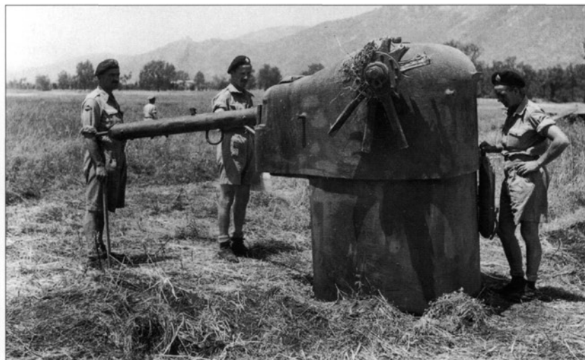
LEFT One of the numerous MG Panzernest , or 'crabs', used in the Hitler Line. This example was captured before it could be buried in the ground. Still attached at the front is the limber and a shattered wheel. The whole structure would have been towed upside down. (Imperial War Museum, NA15778)
