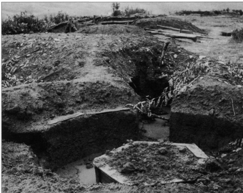
LEFT This field position near Monghidoro formed part of the Gothic Line and was captured by US forces before it could be completed. The trench leading to the dugout is visible at the rear as are the ammunition niches. The pedestal in the middle might have mounted a small anti-tank or anti-aircraft gun. (Imperial War Museum, NA19207)
