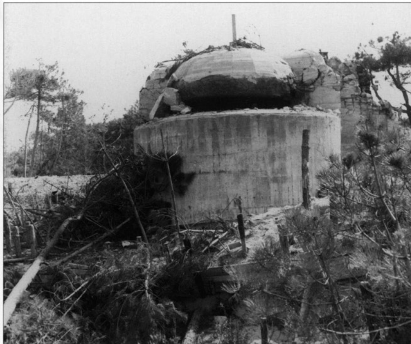
LEFT A destroyed army observation post for a coastal battery (Type 637) that was located on the west coast. In the front section a rangefinder would have been fitted to pinpoint enemy targets for batteries located further to the rear. (US National Archives, 193356)
